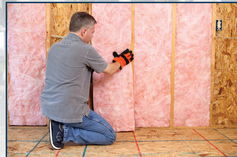
Do it yourself fibreglass insulation installation
